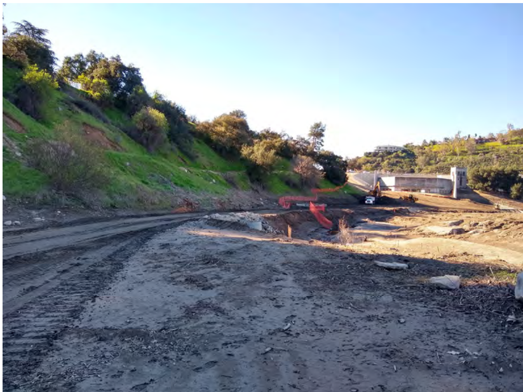
Photograph 2 – West Altadena Drain area after clearing
