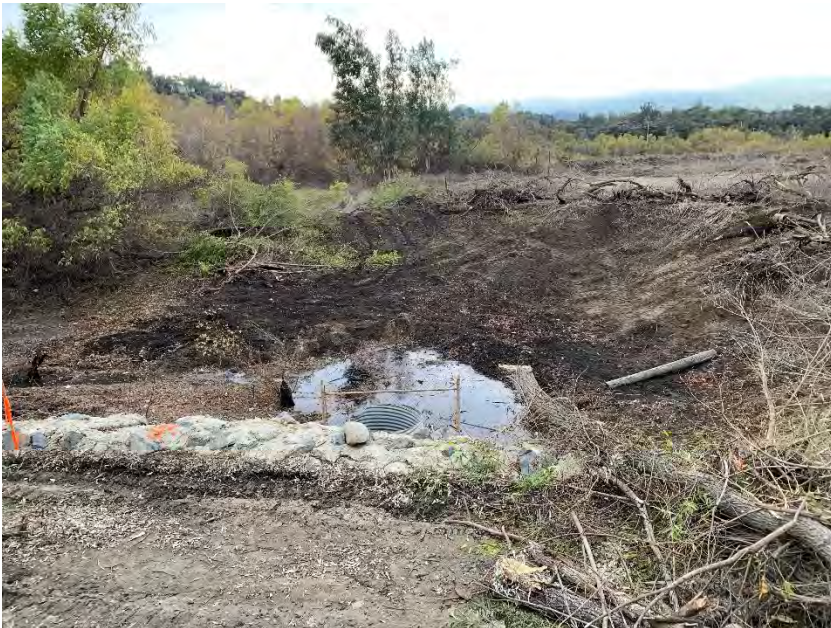
Log Entry #1 Photo D
