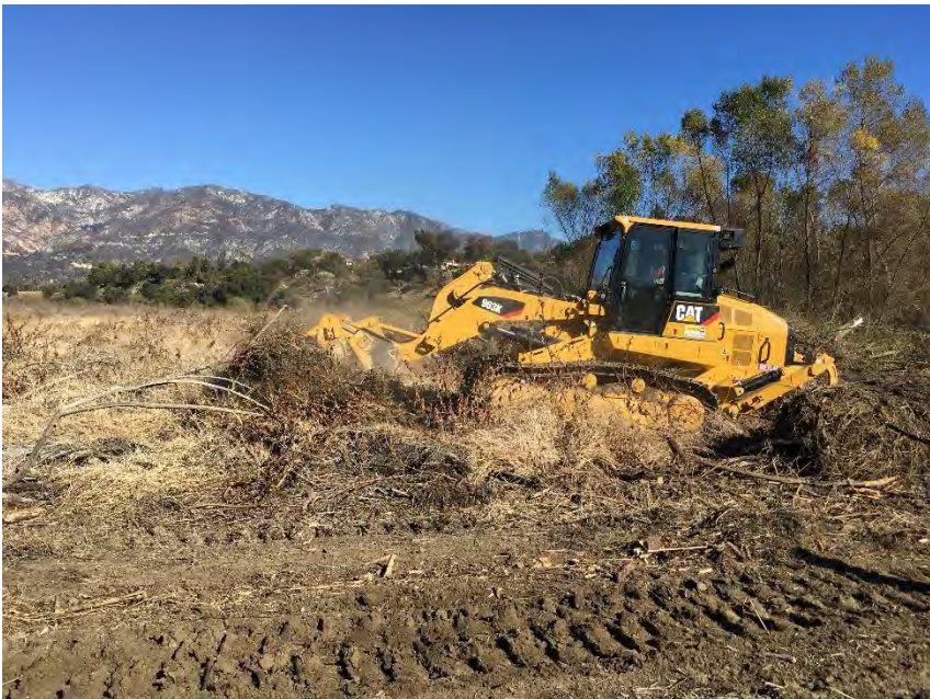
Log Entry #2 Photo D
