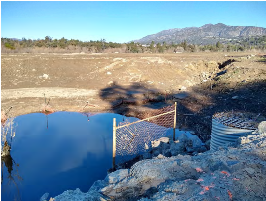
Photograph 4 – West Altadena Drain after clearing
