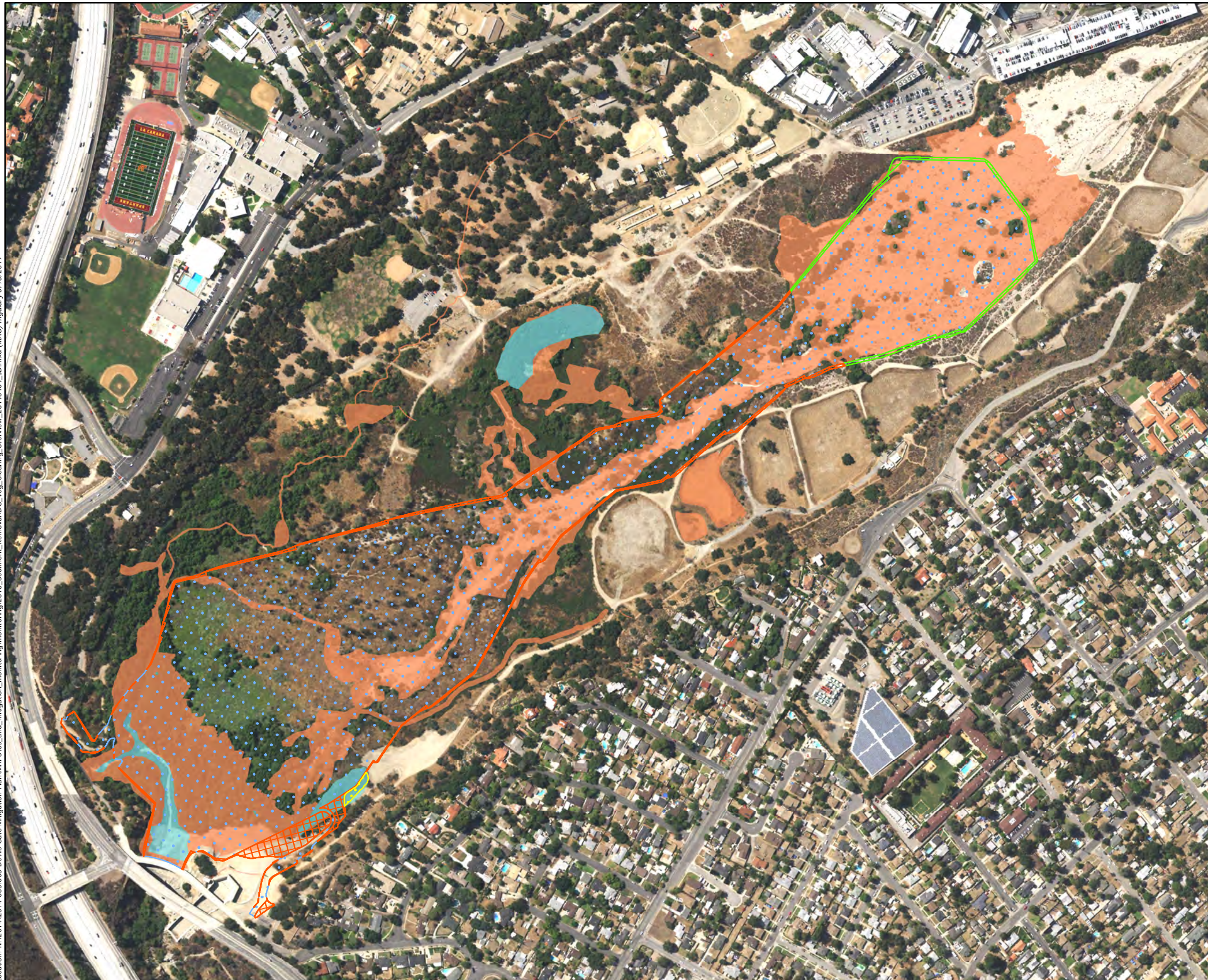
Figure 1. Vegetation Clearing and the Initial Sediment Removal Area
