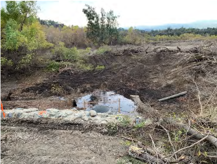
Log Entry #1 Photo D
