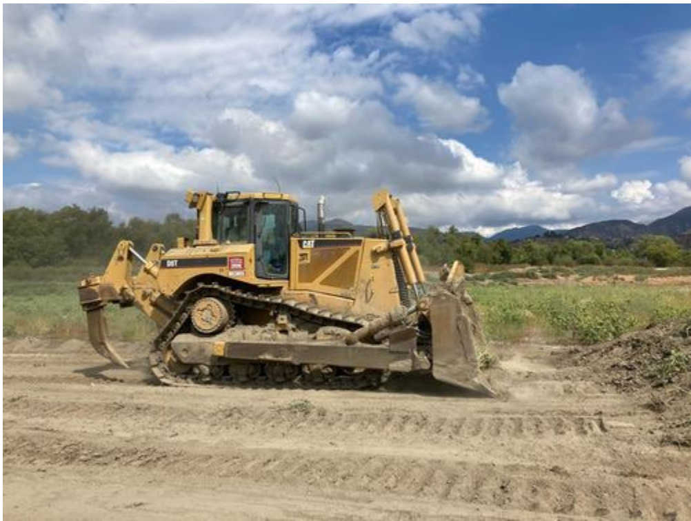
Dozer_continuing_to_remove_vegetation_facing_east.jpg
