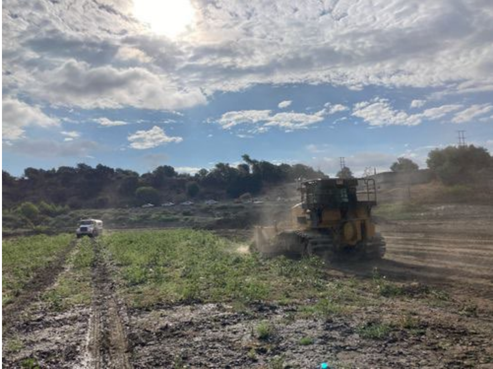
Dozer_removing_vegetation_facing_south.jpg
